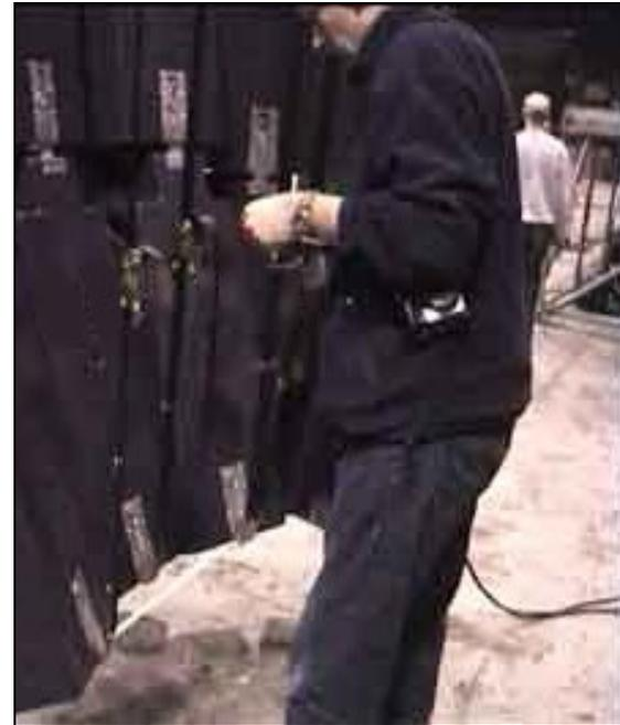
The straps can be hooked into the bottom of the cluster and ratcheted appropriately to ensure a neat array with aligned bottom corners
